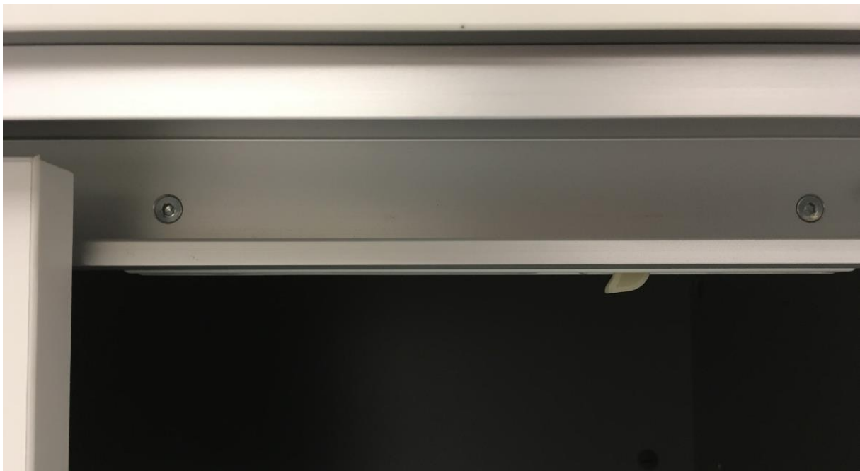
View from the front side: Pendently installed into the sliding door cabinet (1)
